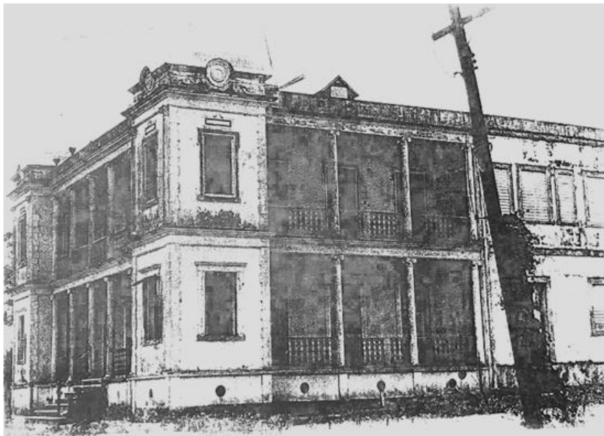
Figure 3.3 Image of the “Castillo Labadie” before its restoration.
