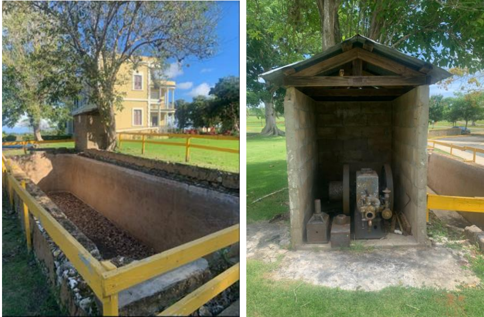
Figure 3.16 The remaining water cistern which originally was covered with a zinc gable roof, just like the one protecting the machinery on the side.
