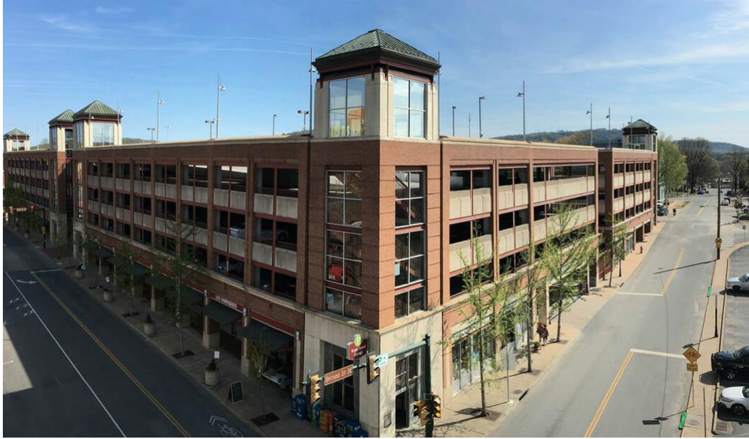
Figure 7. Example of Parking Garage.
