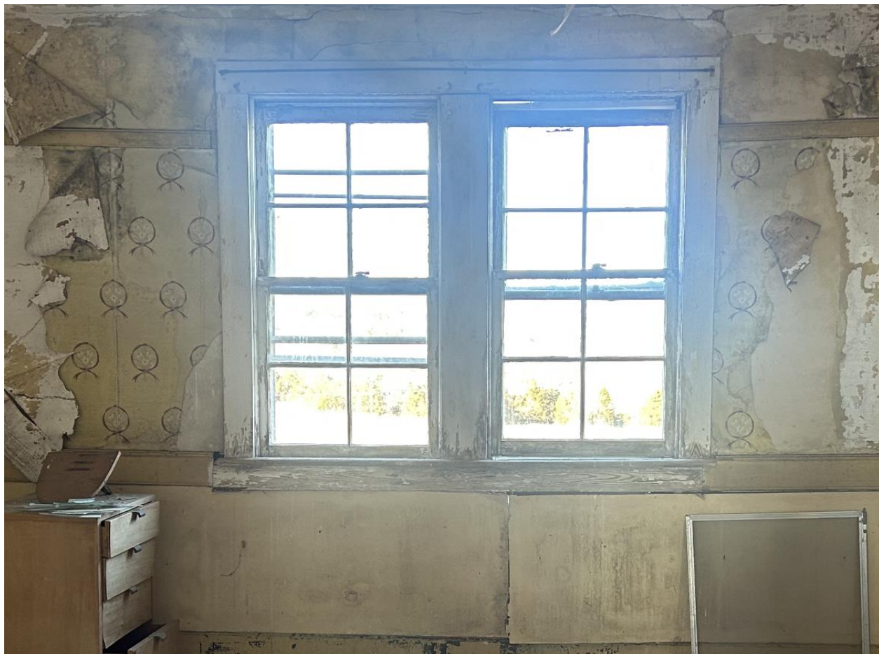
Figure 66: A photo of the double window on the northern end of the second floor of Campaign One. The trim surrounding this window is simpler than the other trims on the second floor.
