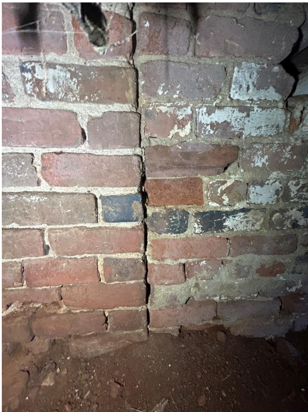
Figure 72: The break in cellar wall between Campaign Two and Campaign Four.
