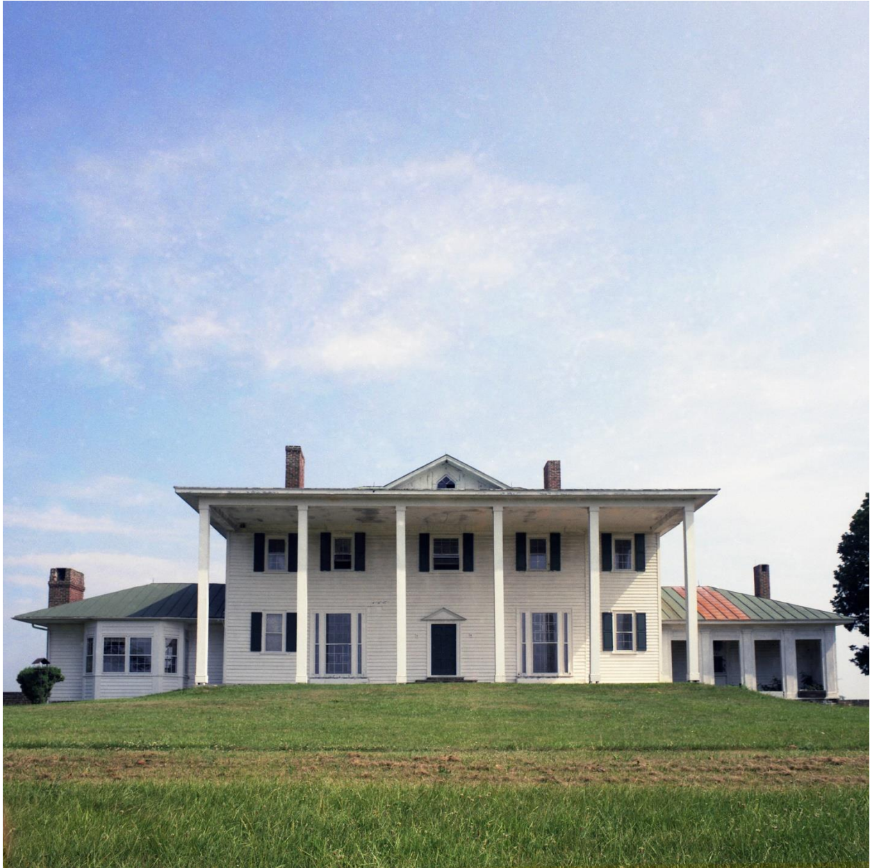
Figure 18: The southern elevation of Sylvania in 1991. Alterations made by Richard Allen shown in this photo include a new porch attached to the main block of the house and a bay window added to the western wing. The grade of the landscaping has also been changed to slope up to the porch addition. Taken by Nancy McEntee in 1991.
