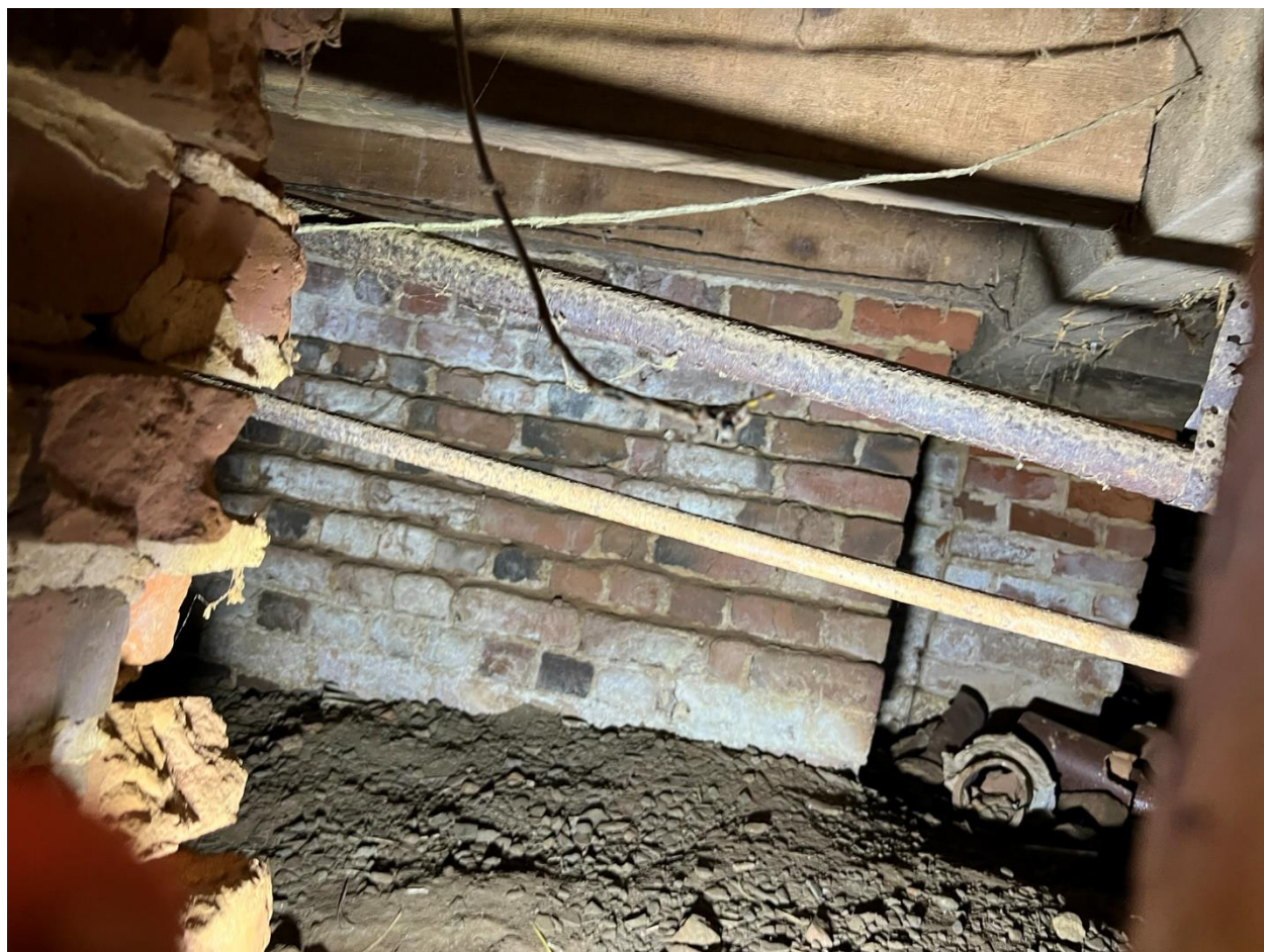
Figure 108: Photo taken from the hole in the west wing, looking into the cellar under Campaign One and Campaign Three. Campaign One's chimney is visible in the background with English bond. Photographed by Will Rourk on March 3, 2025.
