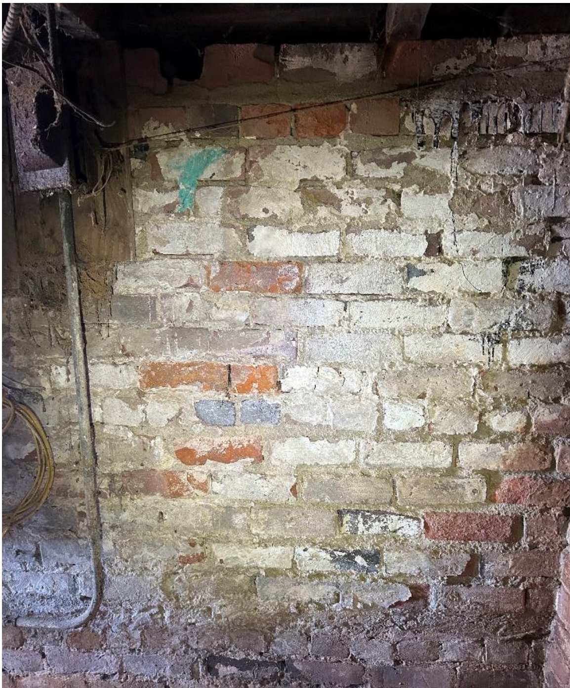
Figure 131: One-to-seven brick bond on the east cellar wall under Campaign Four. This brick bond is consistent on the brick walls dating to Campaign Four.
