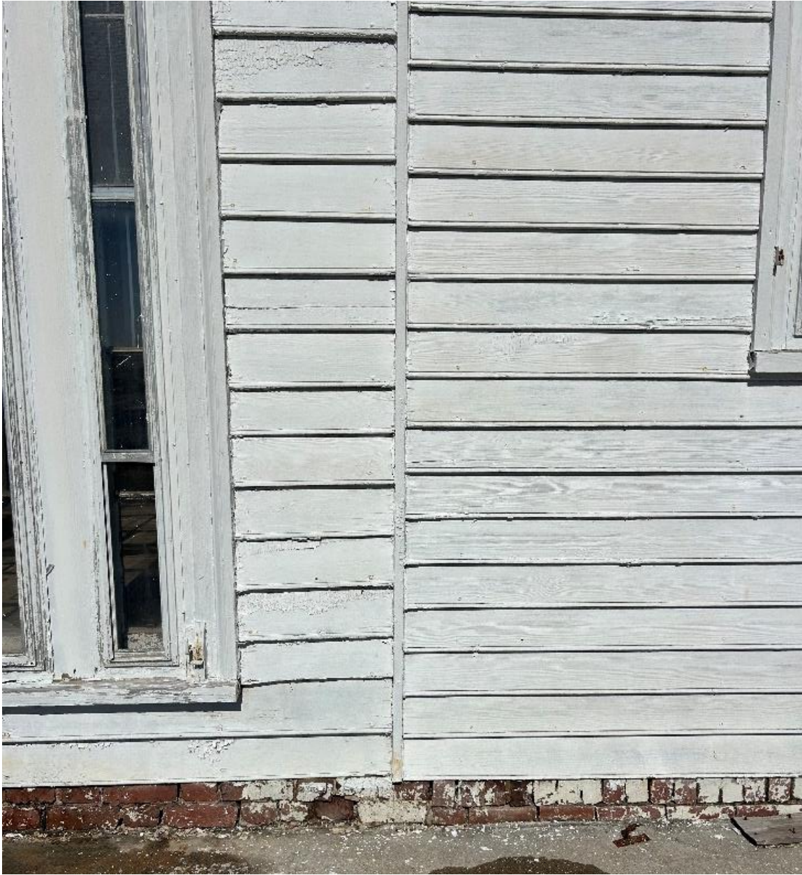
Figure 130: The southern exterior wall where Campaign Two and Campaign Four meet with a visible break in the siding. Below, the brick bond also changes at this point. Both clues indicate that the two campaigns were built at separate times.
