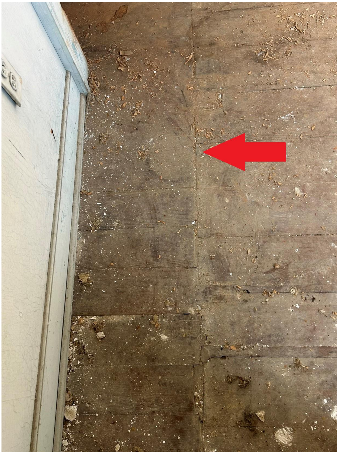
Figure 82: The ghost marks of an old wall are visible where a distinct line in the flooring runs across the floor. The ghost mark of a wall member, seen in Figure 83, is located along this line. This photo was taken in the southeast bedroom in Campaign Two. The ghost marks are adjacent to the evidence for the original stair in the cellar.
