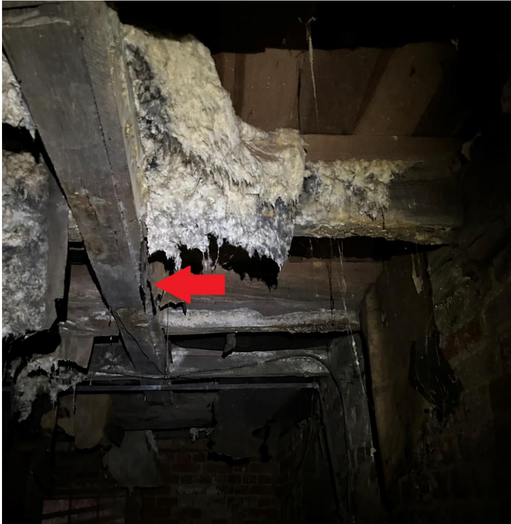
Figure 80: The arrow points to the cross bracing indicating where an original stair was in southeast corner of the cellar in Campaign Two. This bracing is perpendicular to the floor joists, and it is not present in any other location in the cellar. Its location corresponds to the evidence for stairs seen on the second floor. The National Park Service survey also proposed evidence for the outline of the stairs on the brick wall to the right of the bracing, but this evidence is not visible today.
