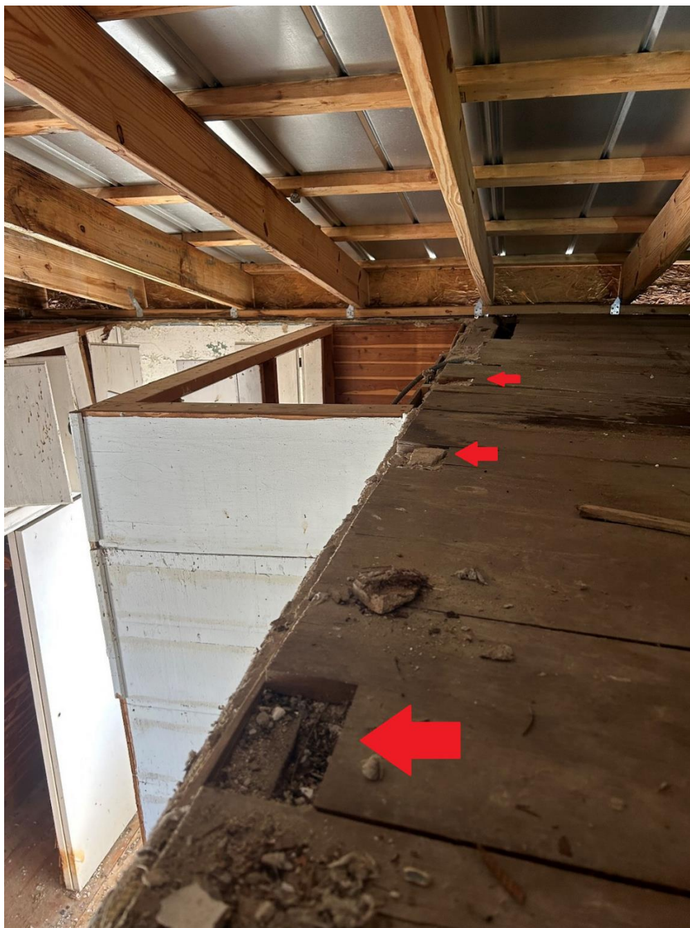
Figure 133: The ghost marks of original roof gable's structural members found on the eastern end of Campaign Two in the attic.
