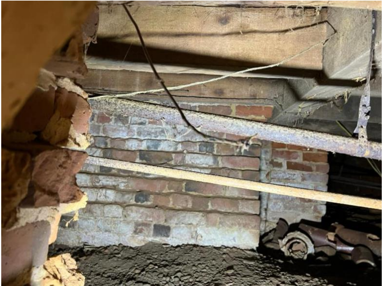
Figure 213: The view of the cellar from the hole in Campaign Five, seen above. From this hole, the base of the chimney, a supporting column, and floor joists are visible. We positioned the scanner carefully to focus on the chimney base and the column beside it. Courtesy of Will Rourk.
