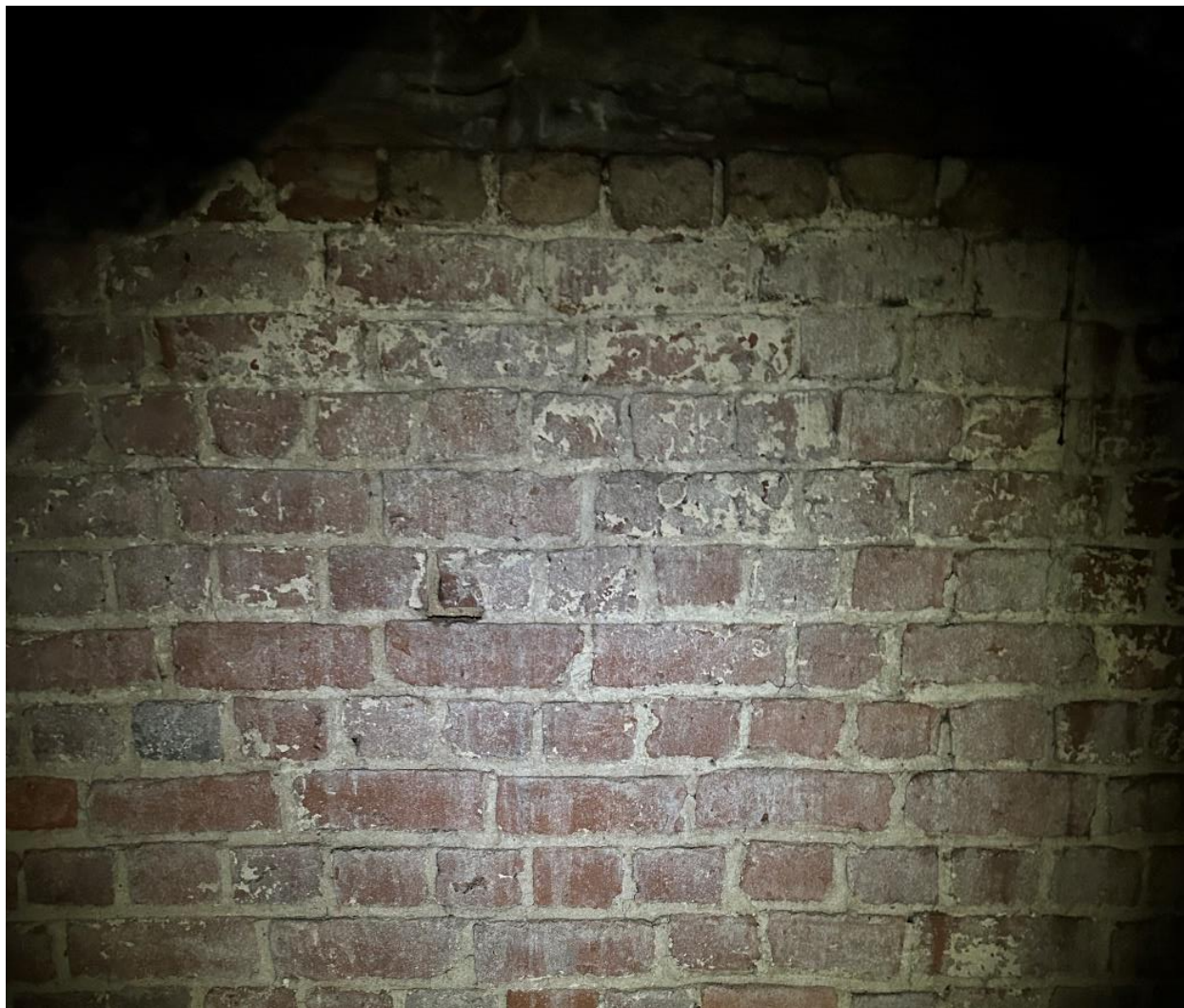
Figure 70: English bond on the southern cellar wall under Campaign Two.
