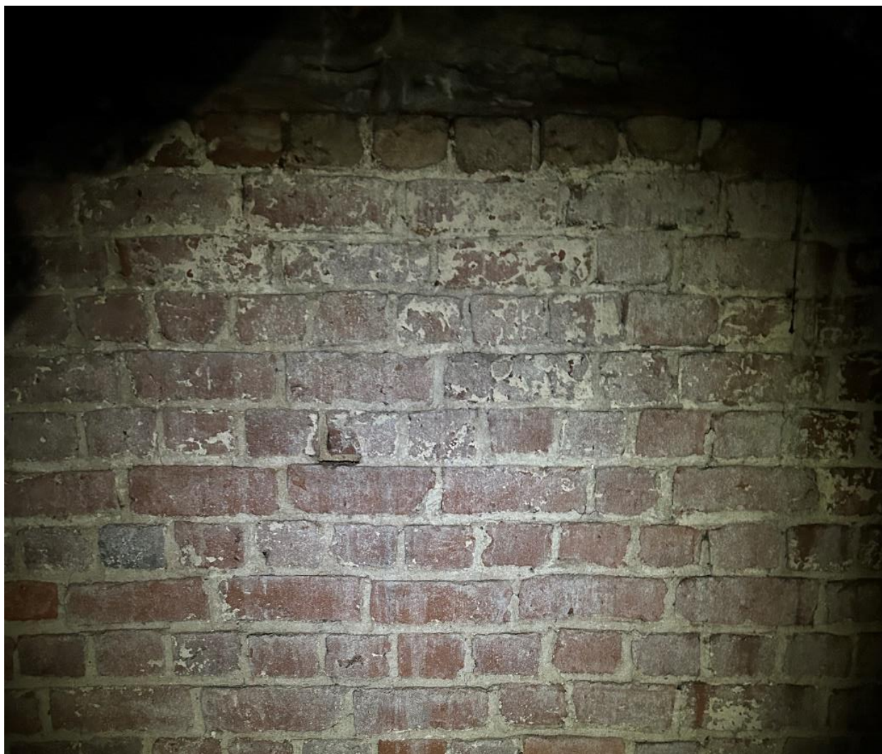
Figure 60: English bond on the southern cellar wall under Campaign Two.
