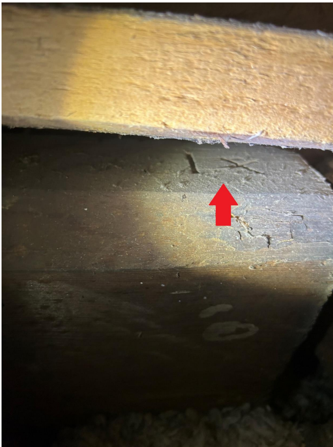
Figure 91: The northern end of the attic where Campaign One and Campaign Two meet with roman numeral “IX”.
