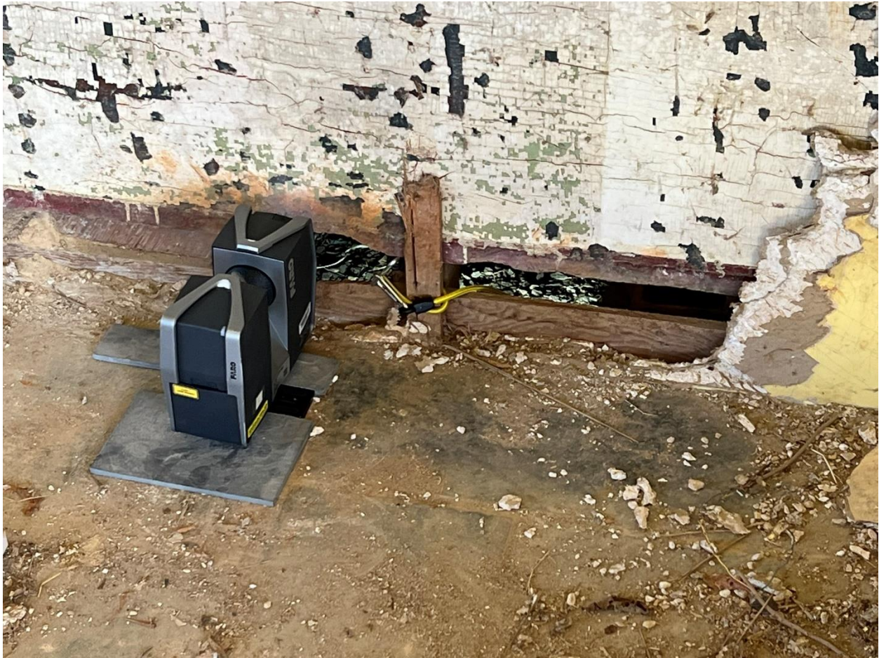
Figure 109: Photo of the hole in the west wing that views the inaccessible cellar under Campaign Three. Two 3D scans were taken from this location to capture the dimensions and location of the chimney base. Photographed by Will Rourk on March 29, 2025.
