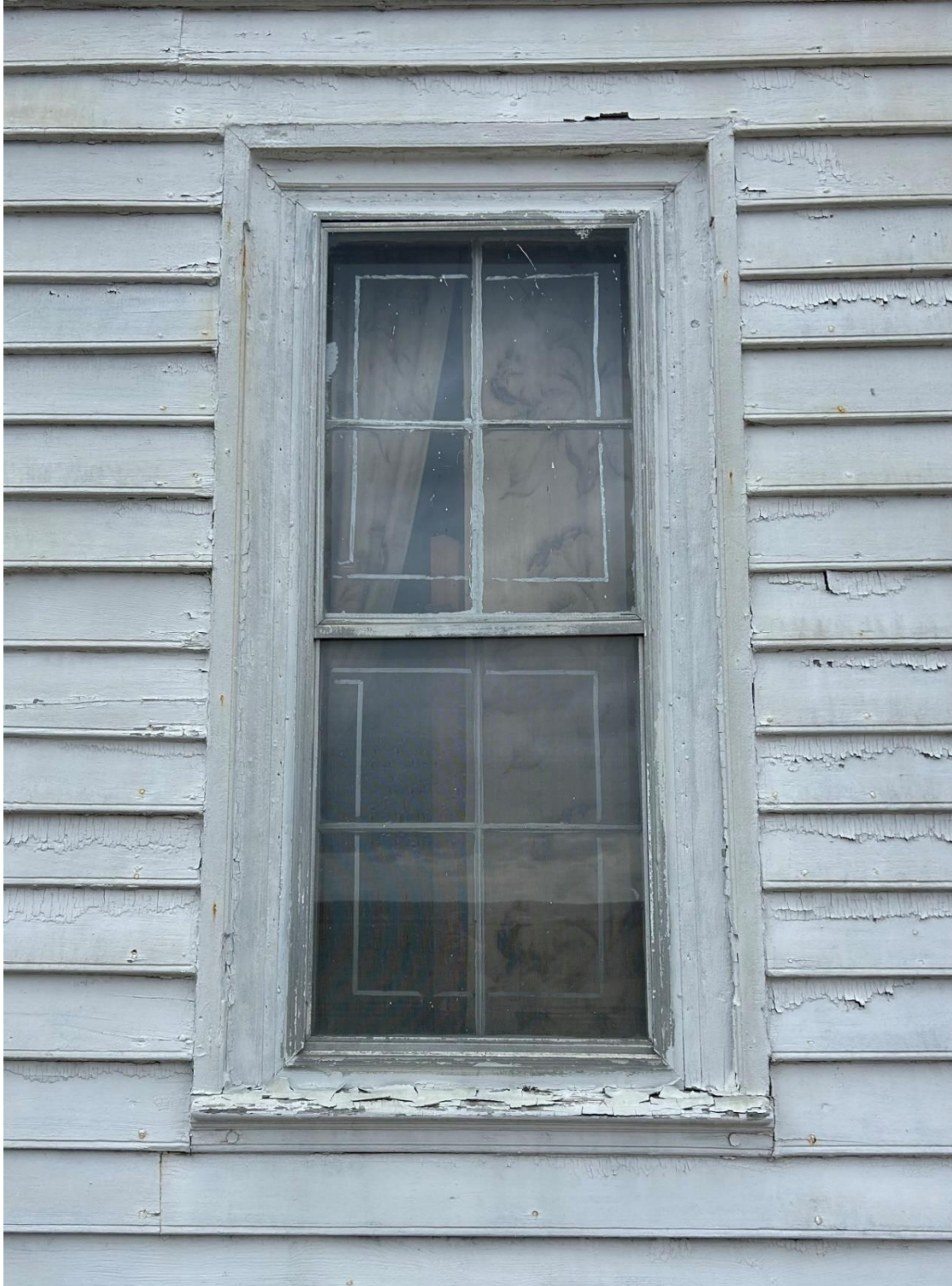
Figure 64: An example of a federal style exterior window trim found on the South elevation, according to Doug Gilpin. This window is in Campaign Three and matches those seen on the second floor of Campaign One and Campaign Two that were highlighted in Figure 63.
