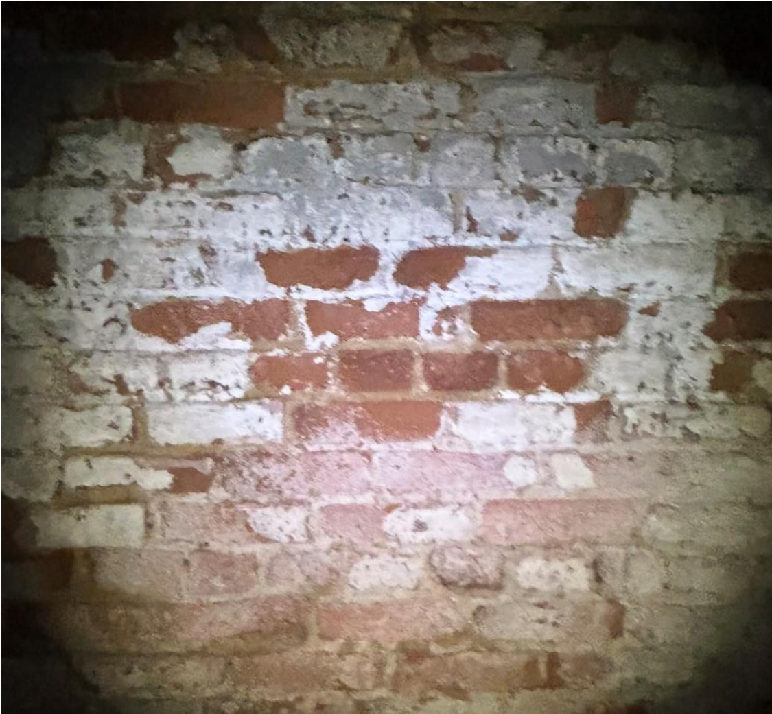
Figure 77: One-to-three bond on the wall dividing the north and south ends of Campaign Two's cellar. This is the only location with One-to-three bond in Campaign Two. It is also seen on the diagonal wall under Campaign One, shown in Figure 114.
