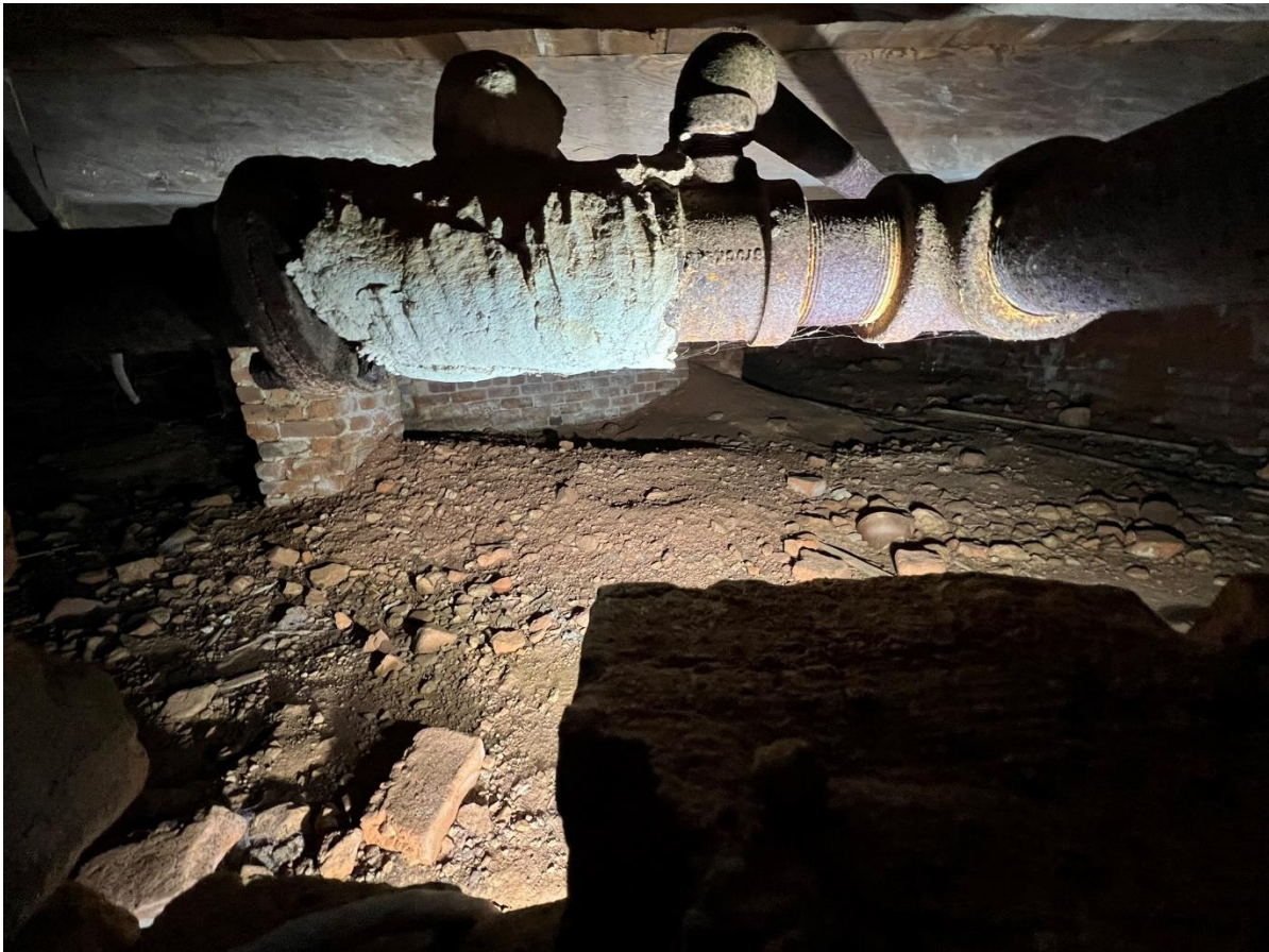
Figure 102: Photo taken from the hole in the cellar wall dividing the cellar under Campaign One from Campaign Two, looking into the inaccessible cellar under Campaign One. The brick column, diagonal brick wall with a One-to-three bond, and the northern wall to the right are visible. Photographed by Will Rourk on March 3, 2025.
