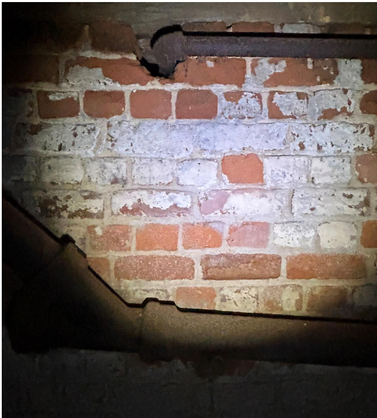
Figure 59: The English bond present on the cellar wall separating Campaign One from Campaign Two with a pattern of alternating headers and stretchers.
