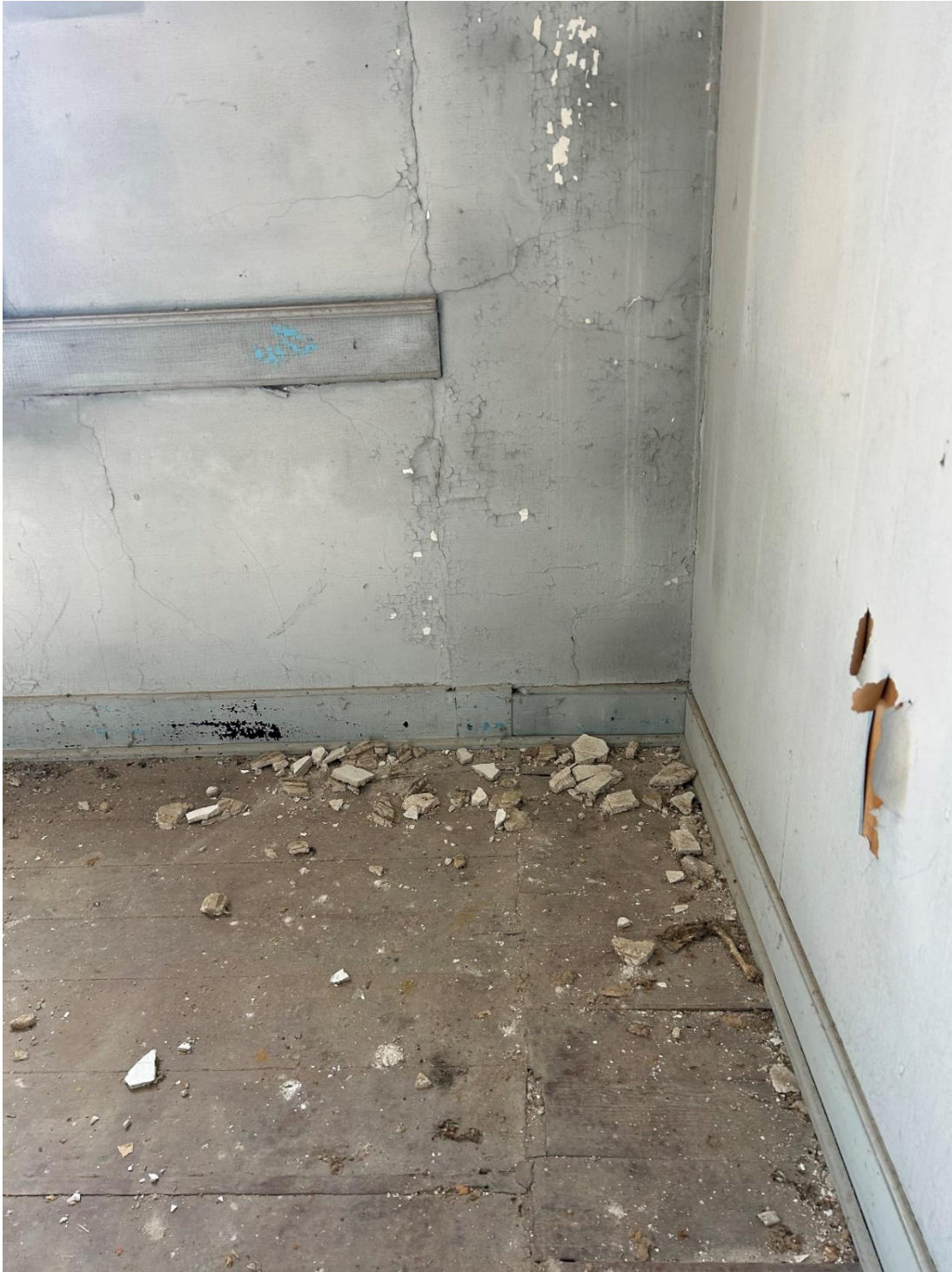
Figure 84: The area where the chair rail stops in the southeast bedroom in Campaign Two that coincides with the ghost marks of an older wall shown in Figures 82 and 83.
