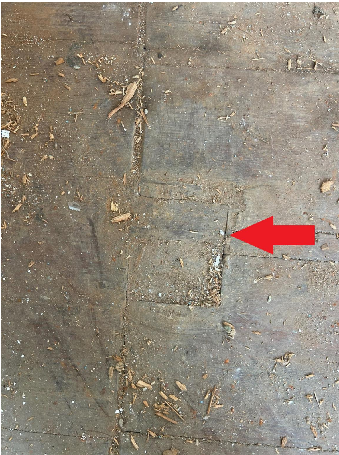
Figure 83: One of the ghost marks of a wall member in the southeast bedroom in Campaign Two that corresponds to the evidence for the original staircase in the cellar.
