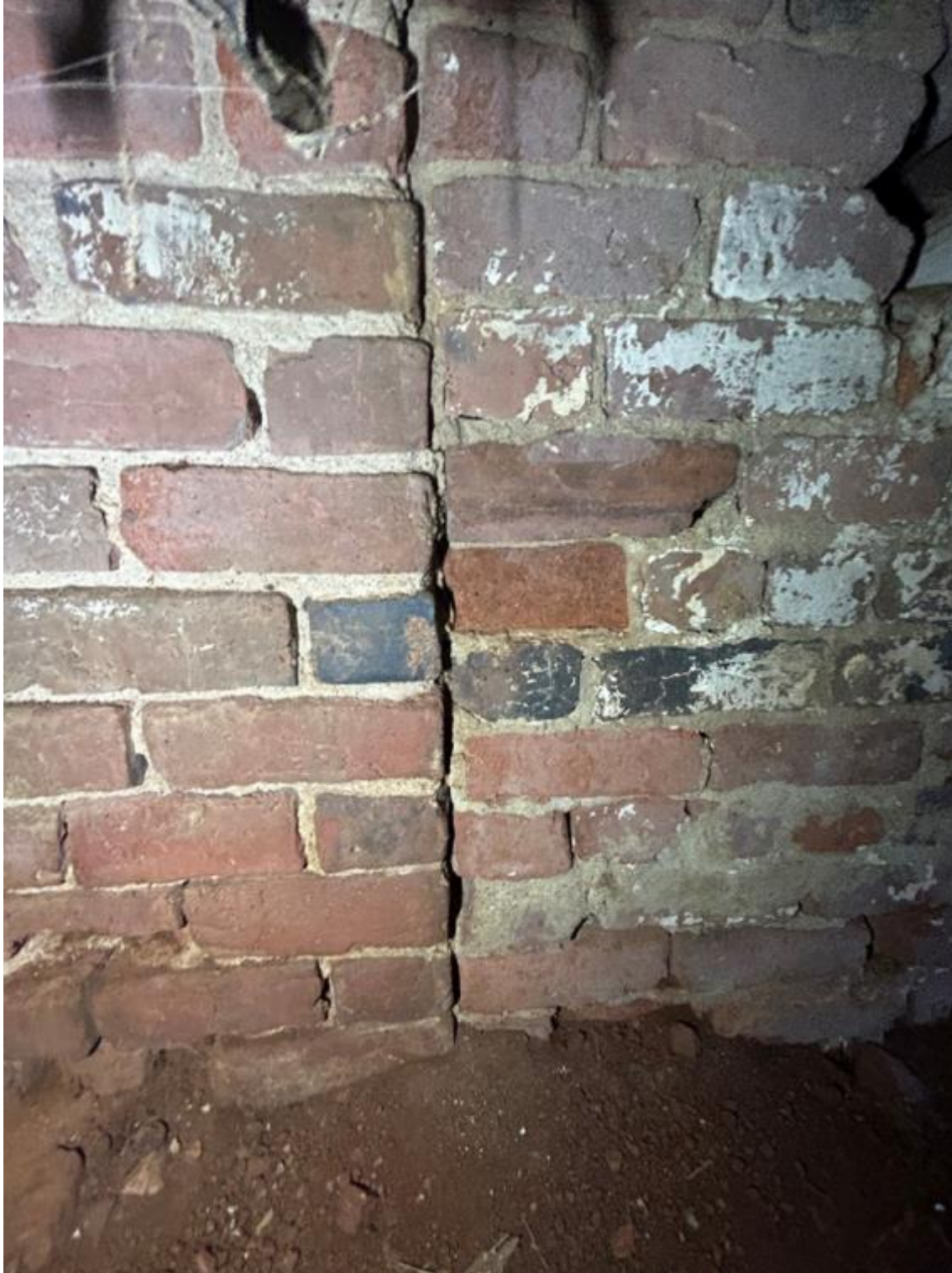
Figure 202: The break in the cellar wall that divides Campaign Two from Campaign Four.
