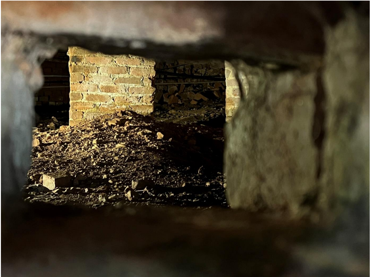
Figure 104: Image of the brick column in the cellar under Campaign One pictured in the center, taken from the hole in the northern exterior brick wall under Campaign One. Behind the column, the back southern wall of the cellar is visible. To the right of the column, the edge of the diagonal wall with one-to-three bond is visible. Photographed by Will Rourk on March 3, 2025.
