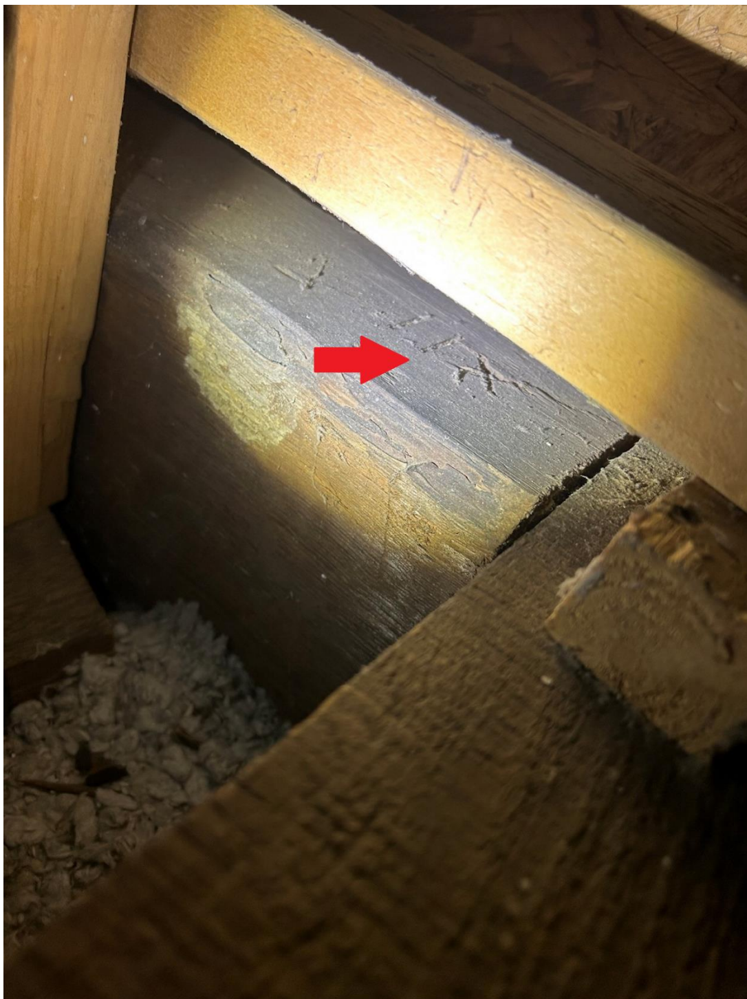
Figure 90: The northern end of the attic where Campaign One and Campaign Two meet with roman numeral “IIX”.
