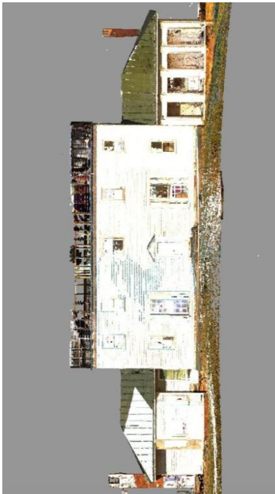
Figure 144: A view of the south elevation of the main house. From this view, the joist information in the attic is visible. This information appears here because our scanners were not placed high enough to capture 3D data from the top of the roof, and we did not have the equipment to do so.
