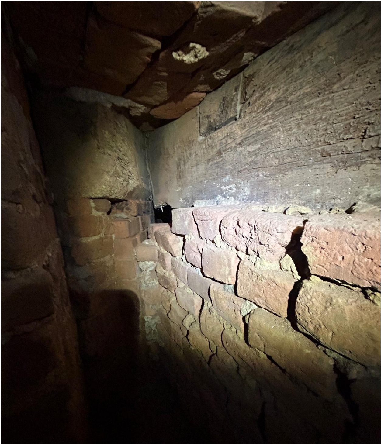
Figure 112: Photo taken inside the cavity under the hearth in Campaign One. The diagonal wall with One-to-three bond that is seen in the 3D scan data is to the right, and to the left is the wall supporting the corner chimney.
