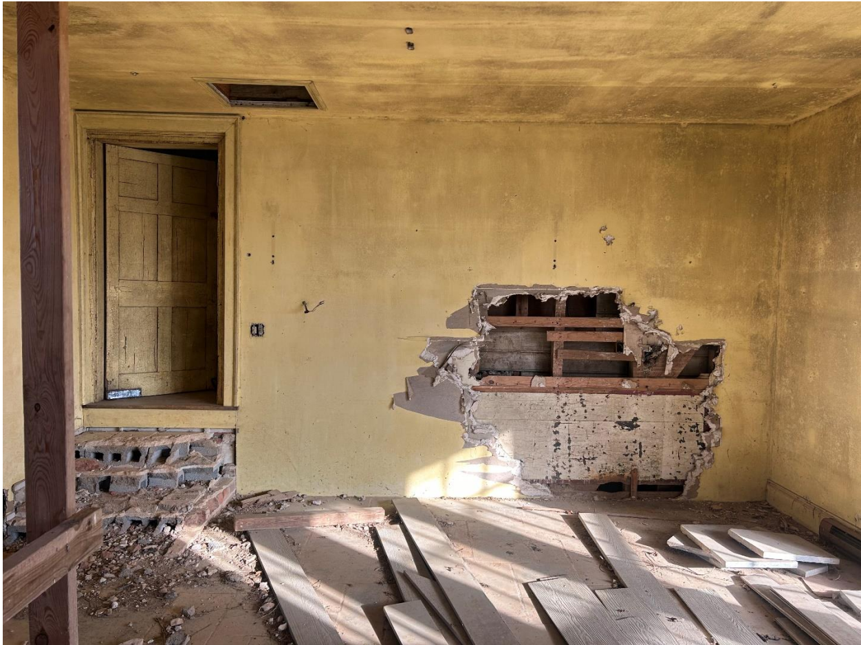
Figure 126: Photo of the hole in the west wing that reveals Campaign Five's original wainscot preserved under the drywall and Campaign Three's exterior siding behind Campaign Five's structural members. This hole reveals how Campaign Five is built against the exterior of Campaign Three.
