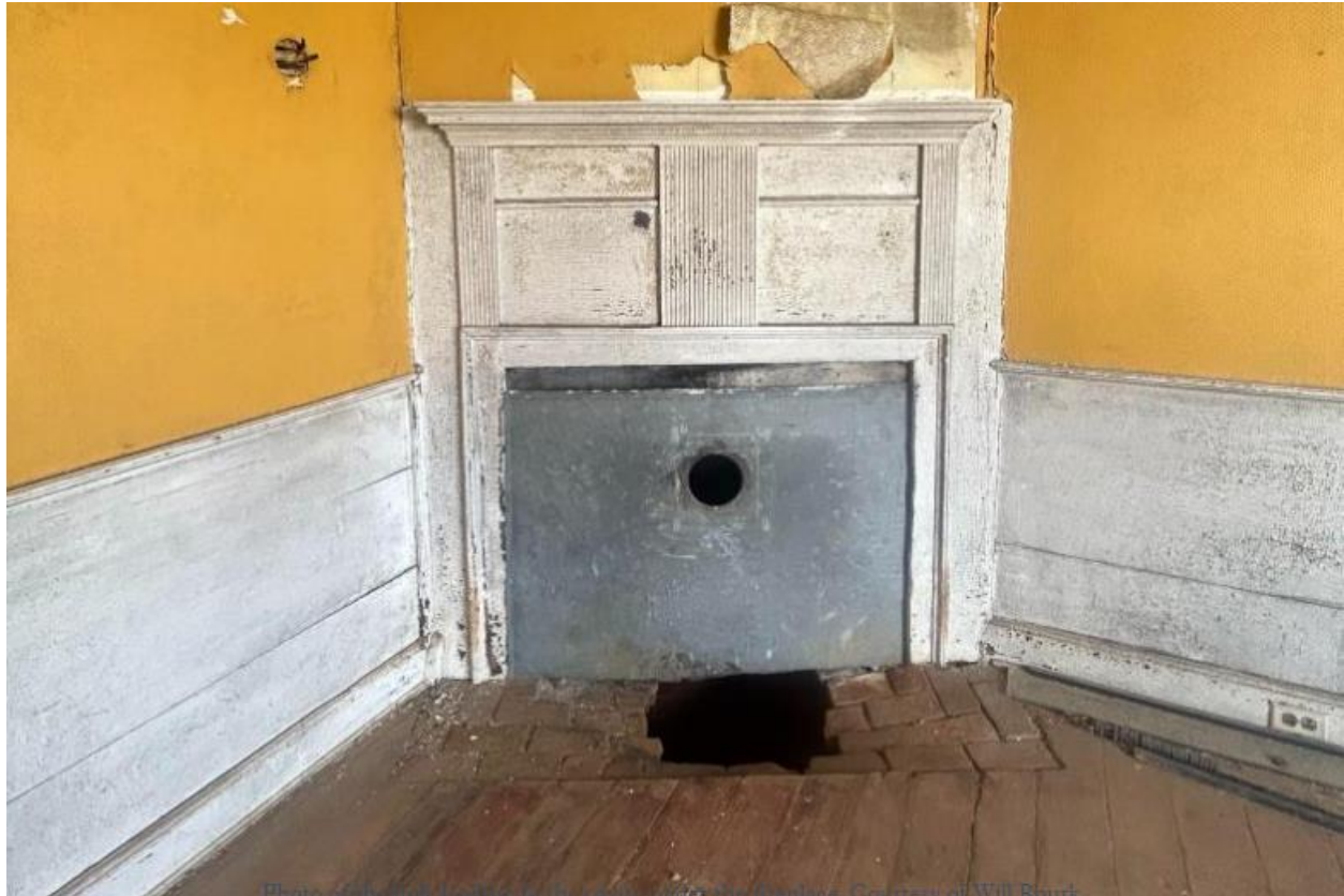
Figure 207: The hole in the floor under one of the corner fireplaces.
