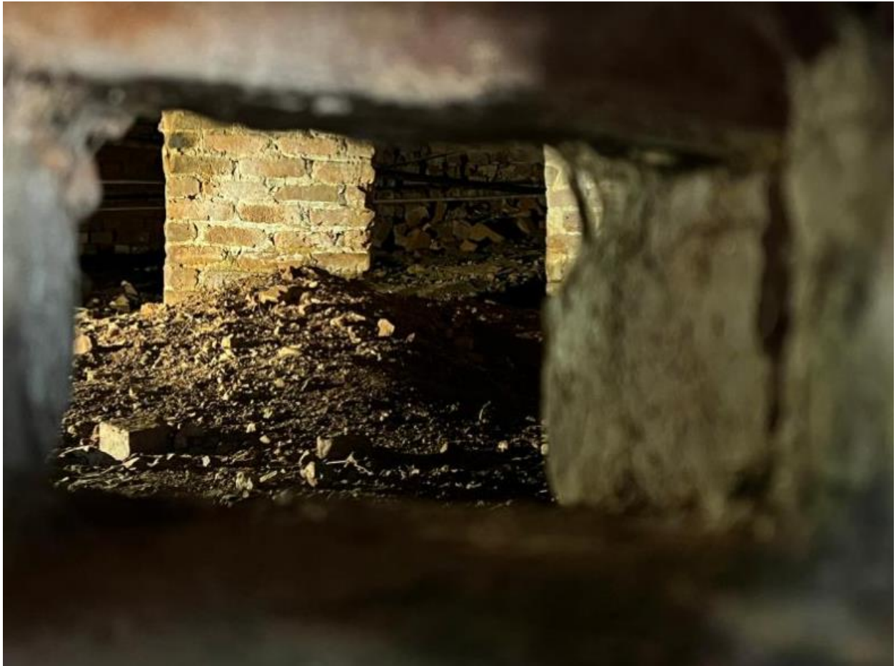
Figure 215: The view from the hole in the exterior brick wall, seen above. A supporting column, the edge of the chimney base, and the back cellar wall are visible. Courtesy of Will Rourk.
