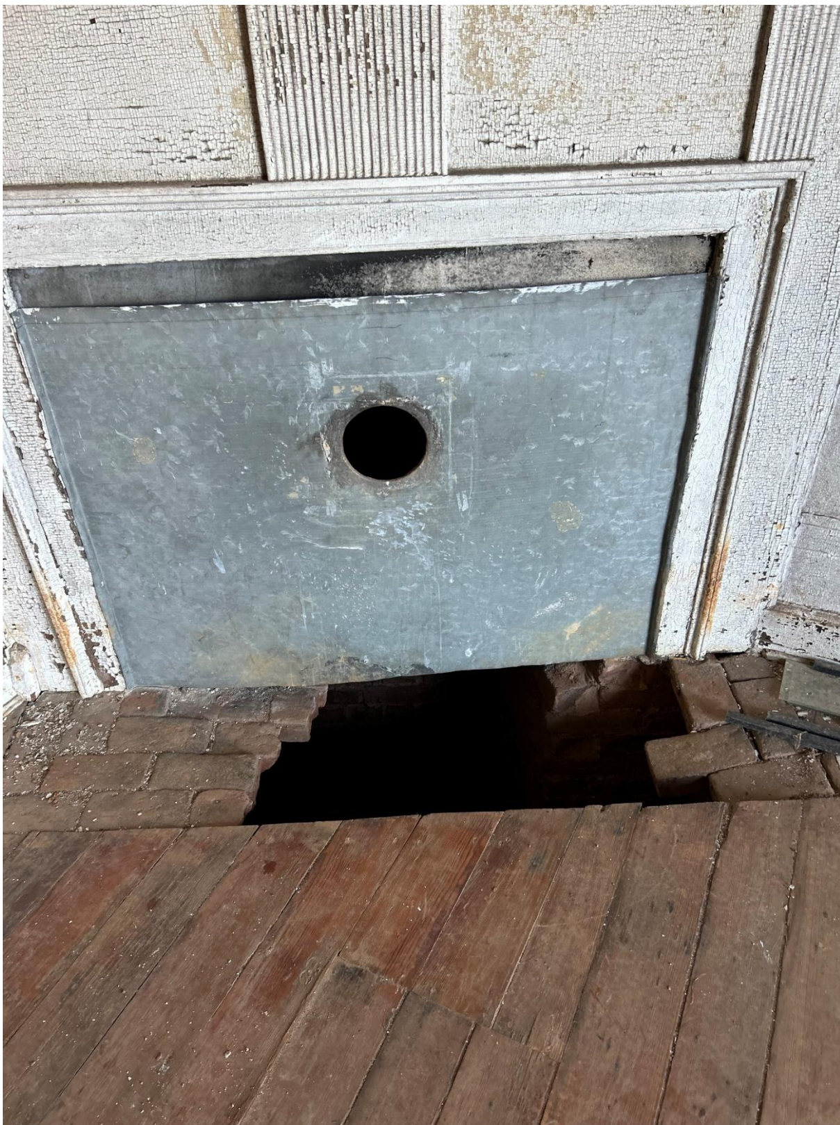
Figure 111: The location of cavity under the hearth in the first-floor northern room of Campaign One.
