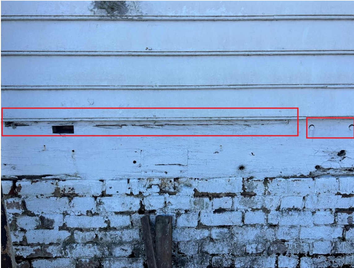
Figure 86: The door sill and pegs visible on north elevation sill plate that indicate the location of the original northern exterior door.
