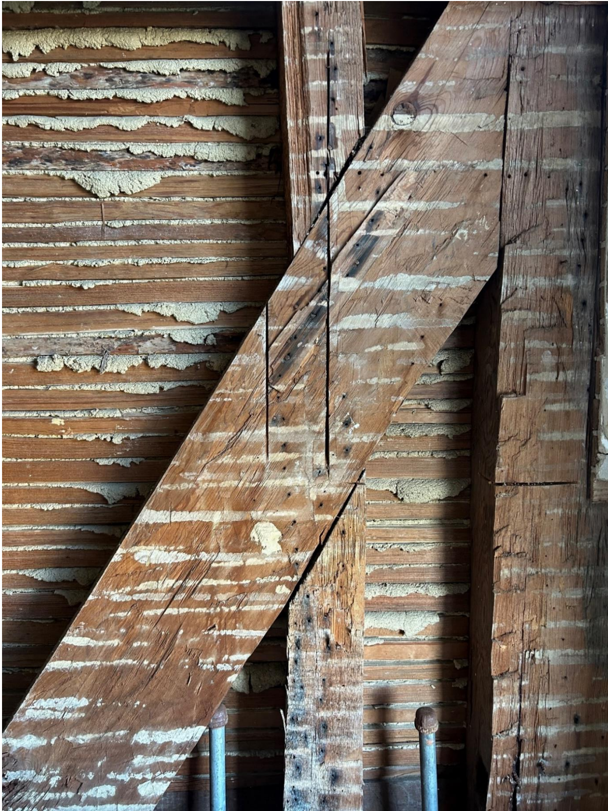
Figure 55: Photo of structural members on the second floor dividing Campaign One and Campaign Two. According to Mark Kutney, there is evidence for mortise and tenon construction joining the cross brace.
