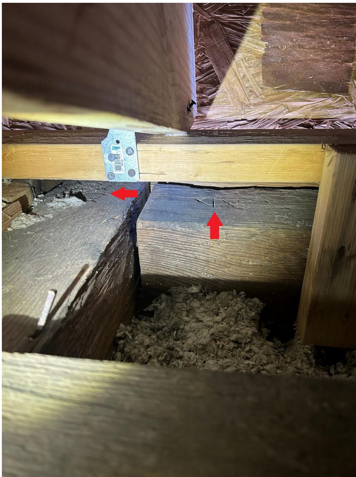
Figure 92: The original northwest corner of the attic in Campaign One with roman numeral “XIX”.
