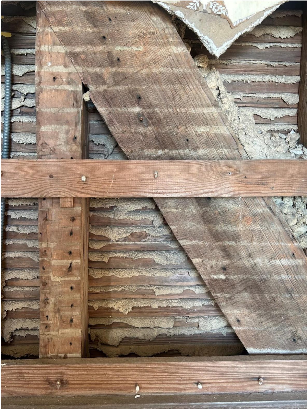
Figure 57: A photo of the visible structural members on the first-floor wall of Campaign One that divides its two rooms. The cross brace is the diagonal wood member in the photo.
