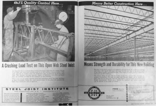
Figure 4.2 - Advertisement for mass produced open web warren trusses. Image from *Architectural Record*, 1958.
