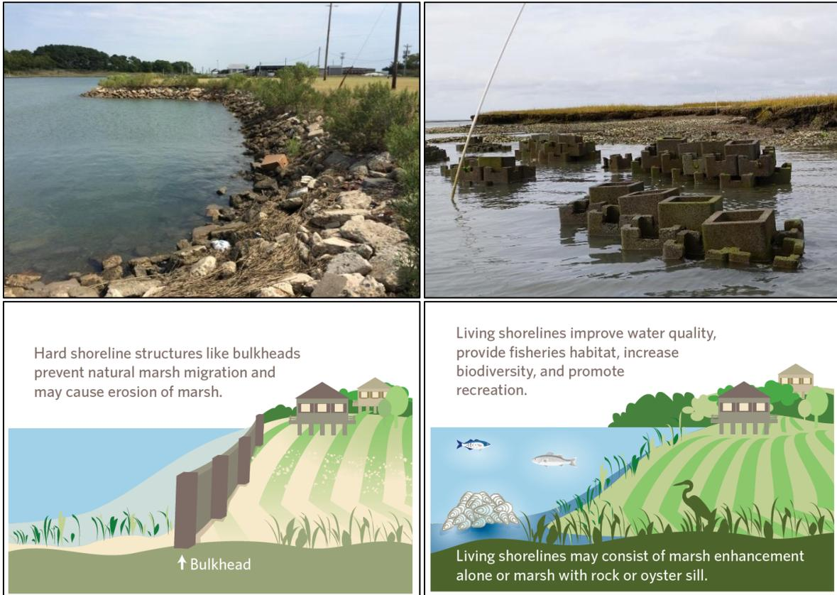
**Figure 1.1.** Hardened shoreline constructed of stone revetment in Oyster, VA (*upper left*) (author). Living shoreline treatment constructed with Oyster Castles® at Man and Boy marsh, VA (*upper right*) (Lusk, 2015). Schematic of a traditional bulkhead (*lower left*) and of a living shoreline (*lower right*) (TNC, 2017).
