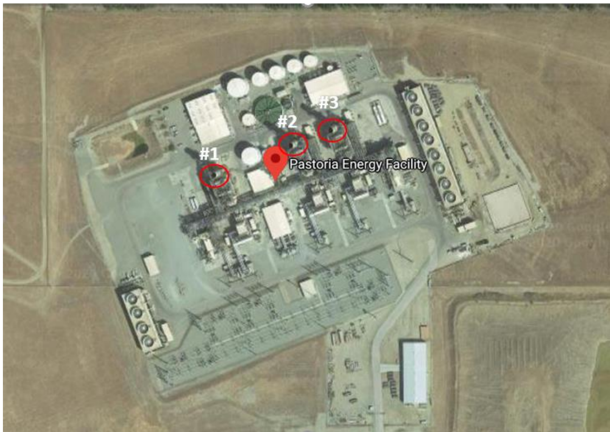
Figure 5: Aerial view of the Pastoria Energy Facility showing each stack.
