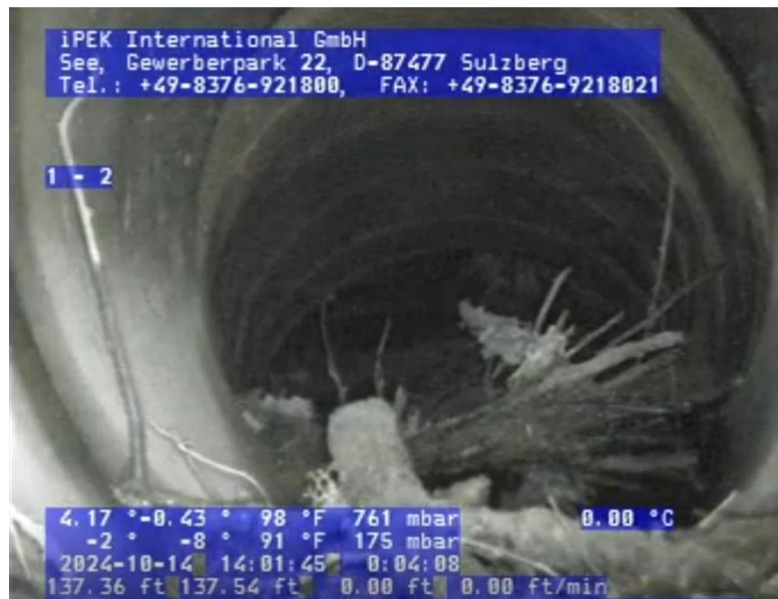
Figure 8: Camera probe image of collapsed pipe
