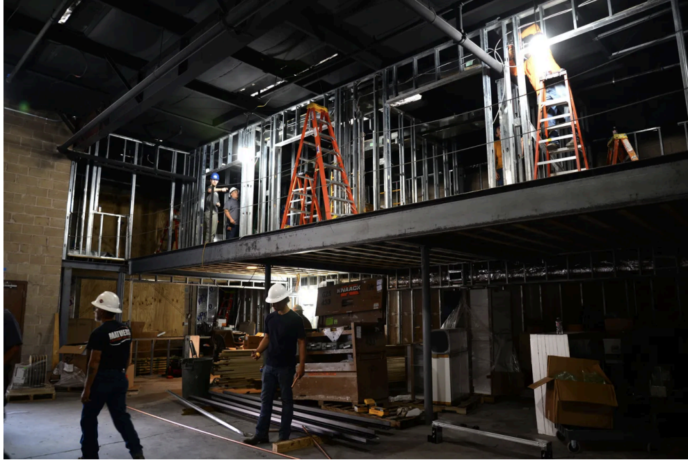
Figure 109: An in-progress photograph of the rehabilitation of the warehouse addition featuring the construction of the mezzanine, 2018. 225
