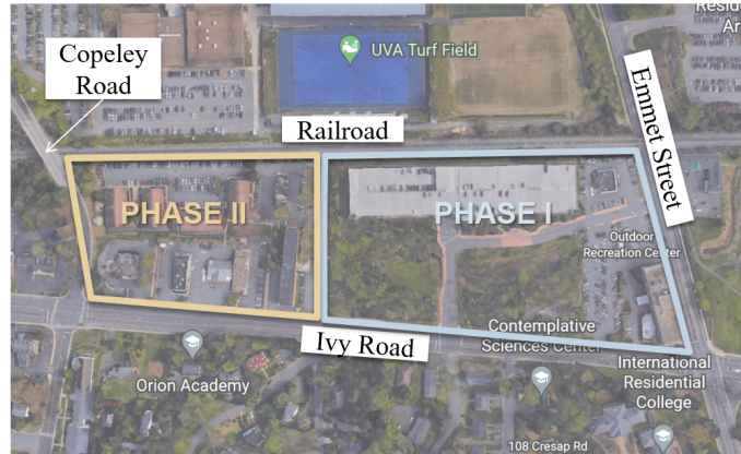
Figure 1. Aerial view of the Ivy Corridor Project with Phase II outlined on the left. Image was captured via Google Earth.
