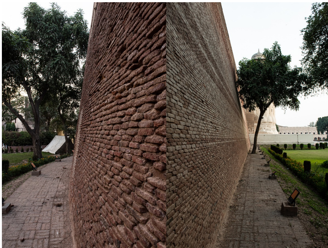
FIG 3.10. Thick buttress walls that form the outer fortification of the Lahore Fort. Picture Credits: M. Farhan Baig
