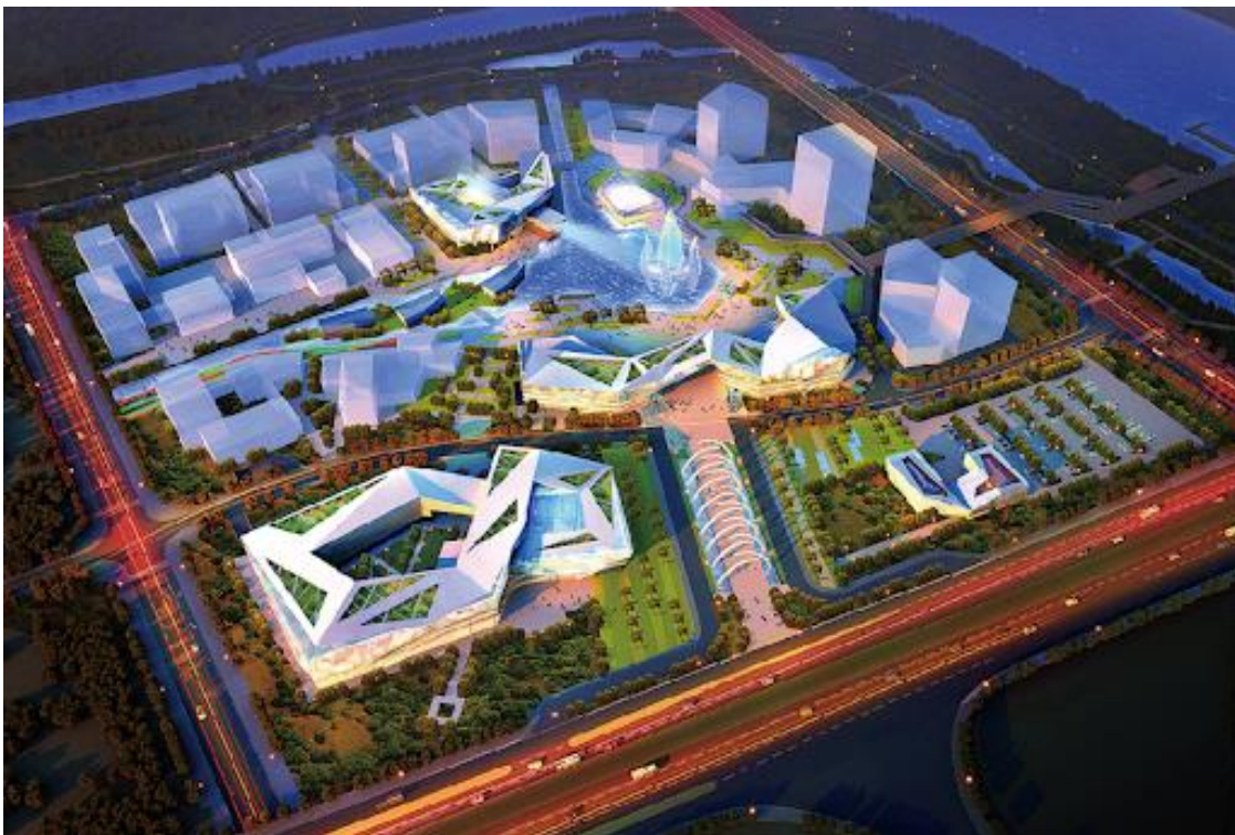
Figure 4: Aerial view of eGamesTown Liangcang Incubator (Reprinted from LC Place , 2020)
