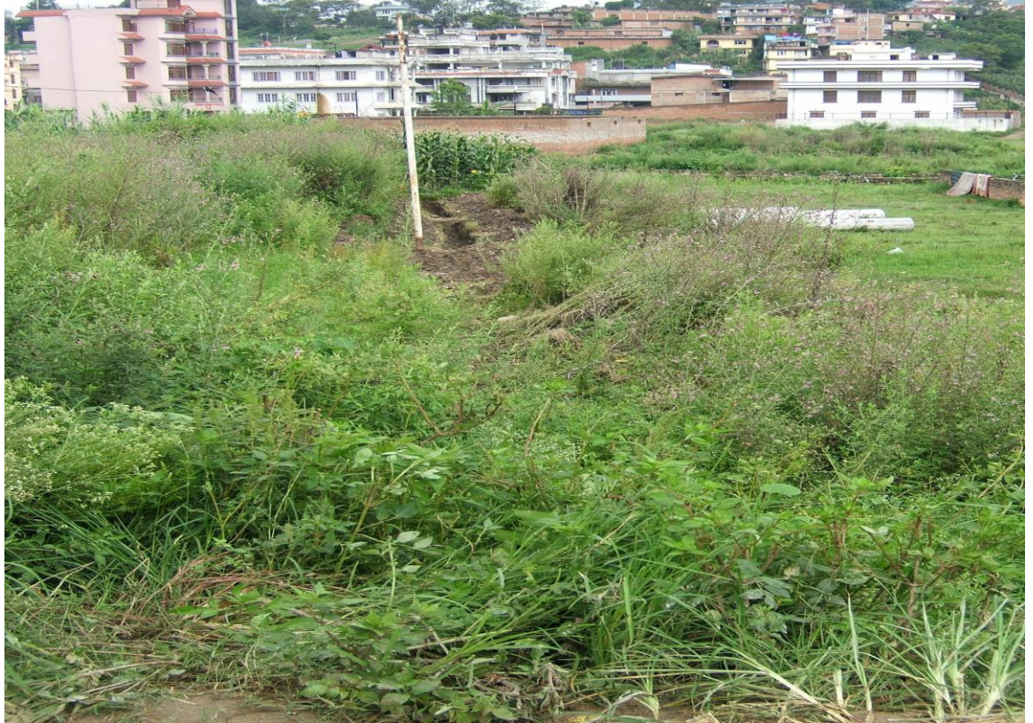
Figure 16. Sewage Line Construction
