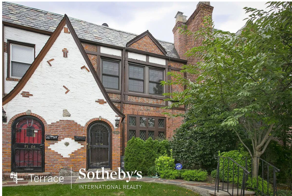
Figure 2-15 Front facade of 91-04 68th Avenue (image from Zillow.com 107 ).
