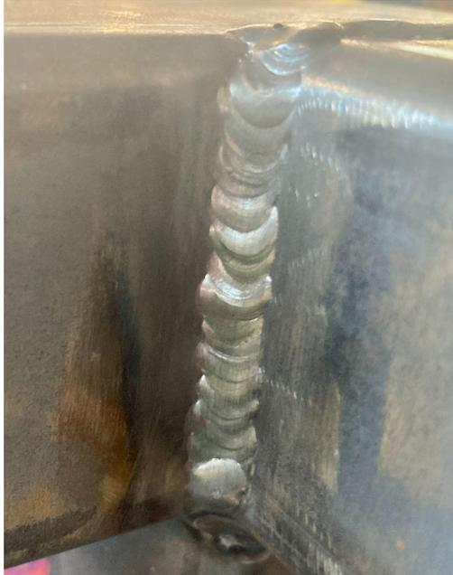
**Fig. 13:** Interior Frame TIG Weld
