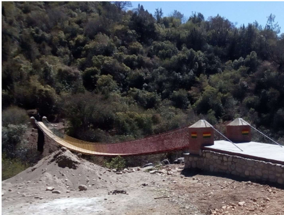
Figure 1. A photograph of a suspended bridge designed by Engineers in Action (Engineers in Action, n.d.).
