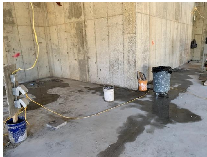
Figure 5. Temporary power station is shown in left side of image (Repak, A., Hussain, A. et al., 2022)
