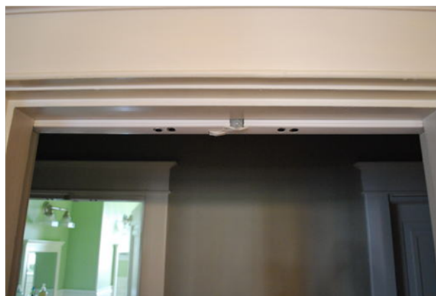
Figure 1.1: Doorway sensors are placed at the top of the doorway and designed to blend in. Sensors face down or out towards the rooms and residents.
