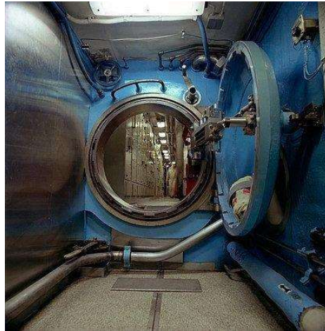
Figure 2: Image of Submarine Watertight Door.
