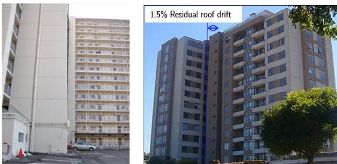
Apartment building with 2% residual drift after the 2011 Tohoku earthquake in Japan [20]
